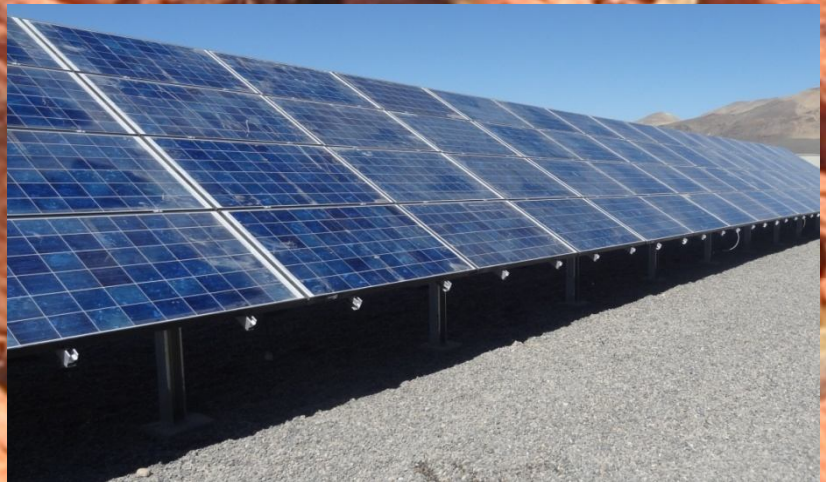
NYTC, 600KW PHOTOVOLTAIC SYSTEM
