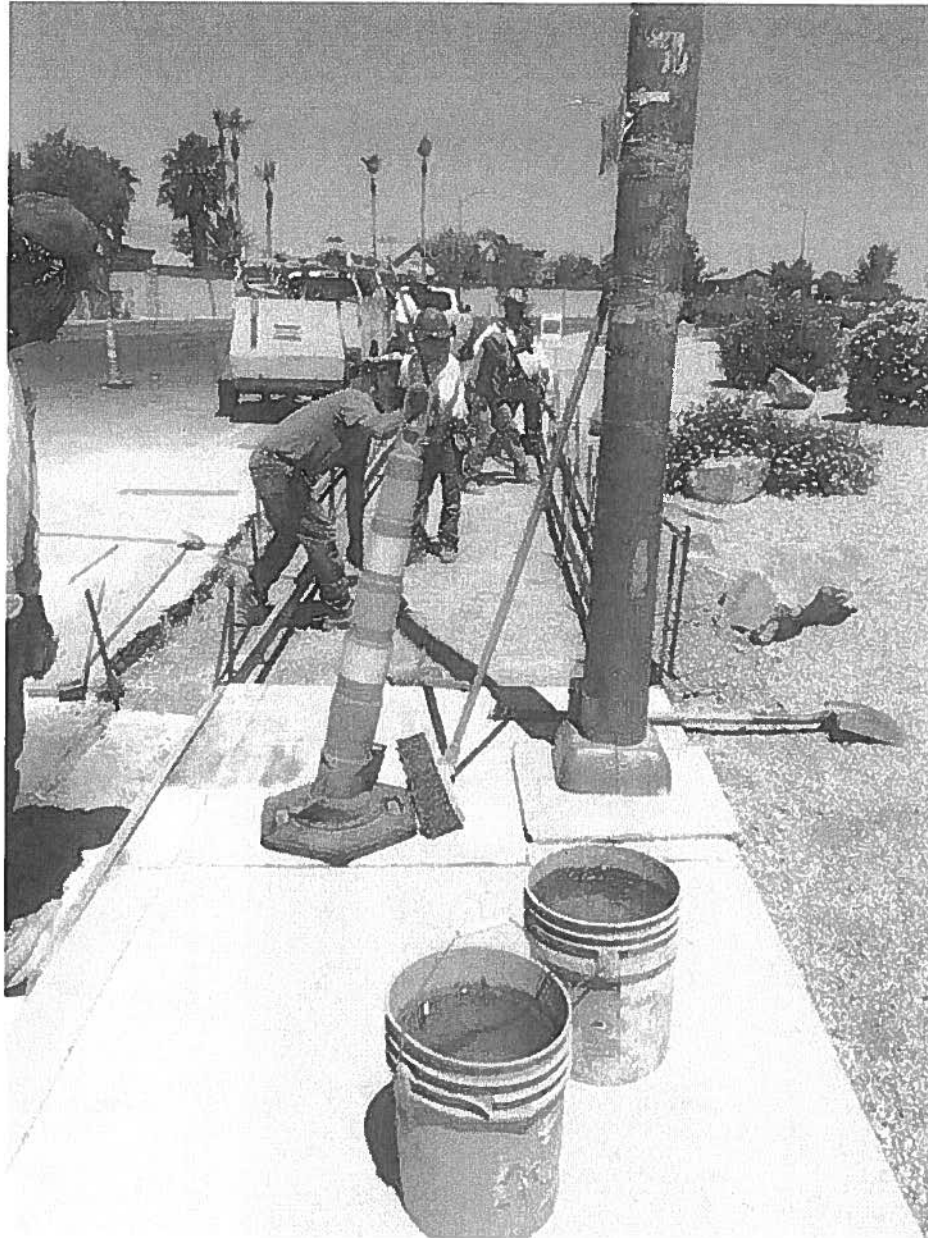
Figure 3 – Installing new ADA ramp for new pedestrian crosswalk at Cimarron Rd./Soaring Gulls Dr. in CLV.
