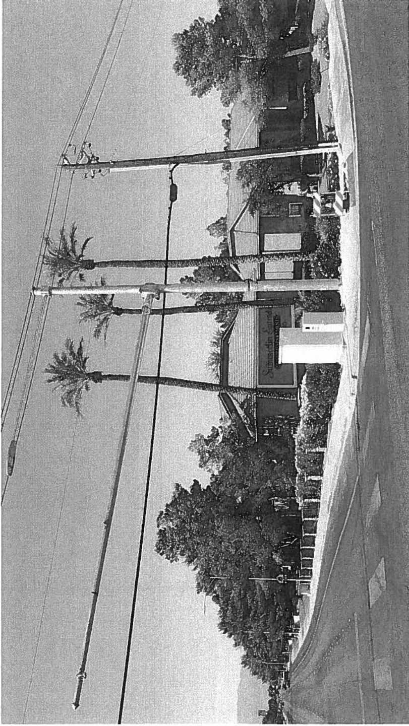
Figure 2 – Installation of push button activated pedestrian signal pole and ADA compliant sidewalk ramp at Vegas Dr./Rock Springs Dr. in CLV
