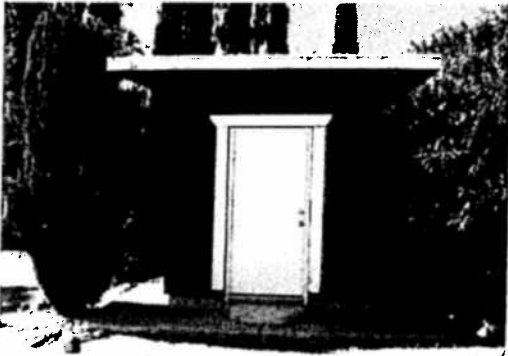
Two views of the utility shed
